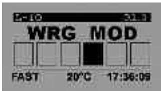
Location of the wrong module in the system (here 3rd module from the right side on a 6-slot cabinet)
