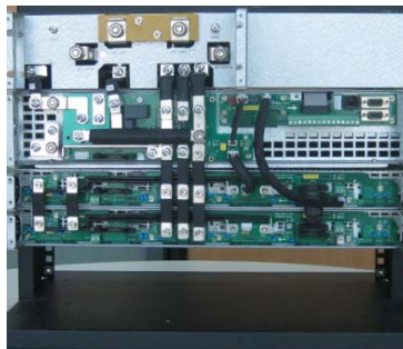
Figure 8–Preparation of the MBS/PD chassis rear cover
