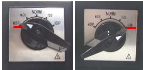
Figure 12–MBS switch positions, MBP or IBP
