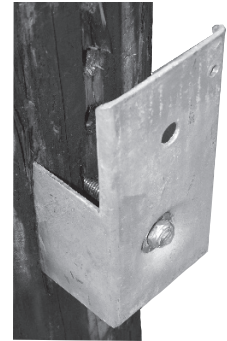
Fig. 2-2, Secure upper bracket
