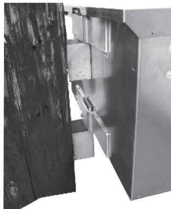
Fig. 2-3, Positioning the enclosure on the pole
