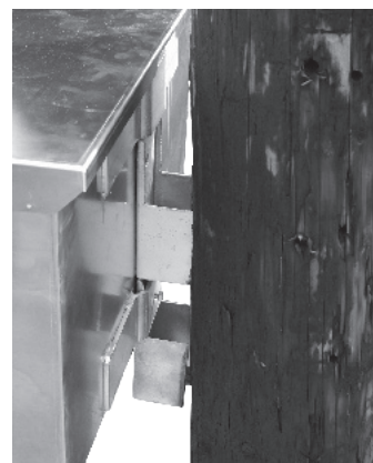
Fig. 2-3, Positioning the enclosure on the pole
